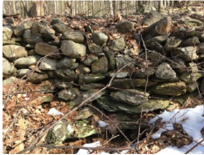
④ Old Stone embankment
