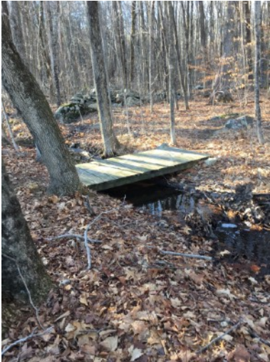
② Bridge crossing the Brook near the Trailhead
