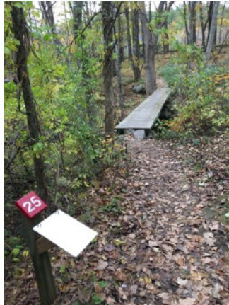
1 Great Brook Bridge
