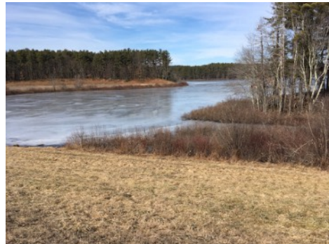
④ Delaney Flood Control Site
